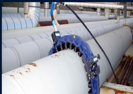
GUIDED WAVE INSPECTION
