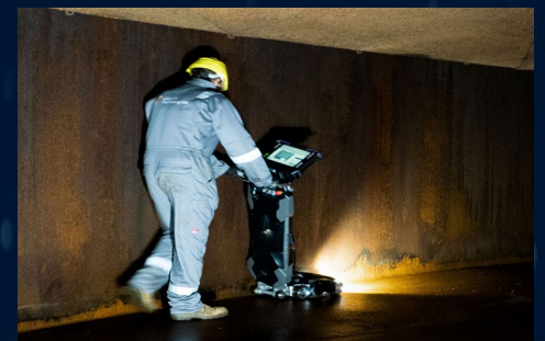
MFL FLOOR SCANNING
